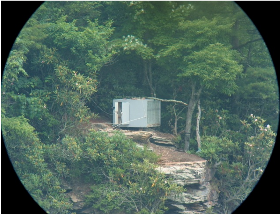
Hack box # 2 (Main hack box) at Grandview from North Overlook
